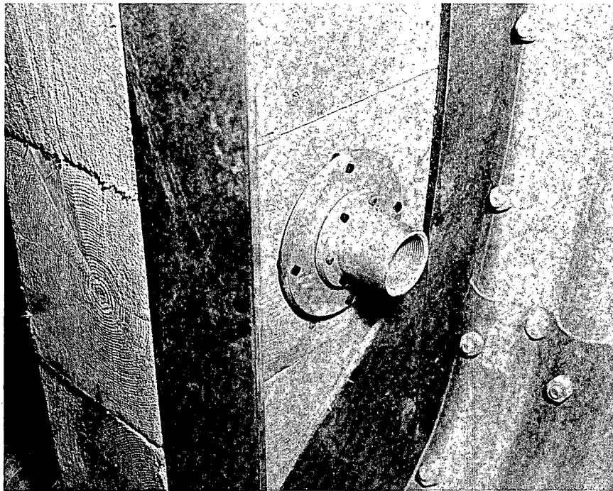
Figure B.6 Peak pressure gage installed on timber bulkhead at access-end of conduit.
